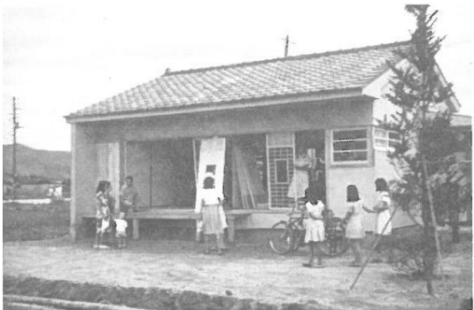
28 Installing the furniture
