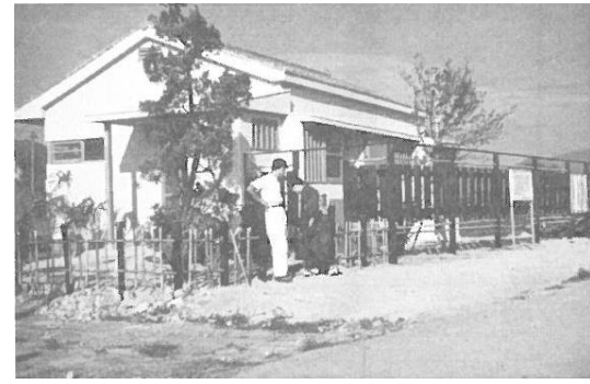
29 Completed show house
