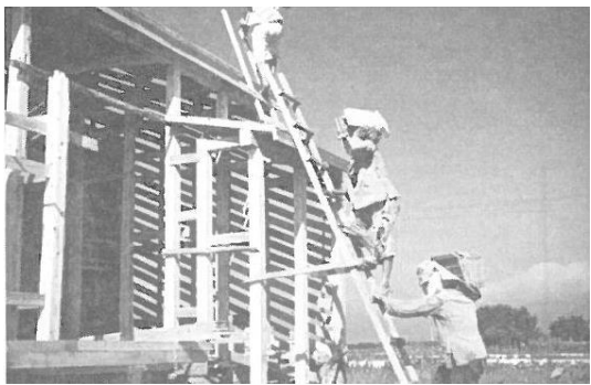
26 Placing tiles on the roof
