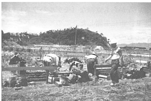
22 Laying bricks for the foundation
