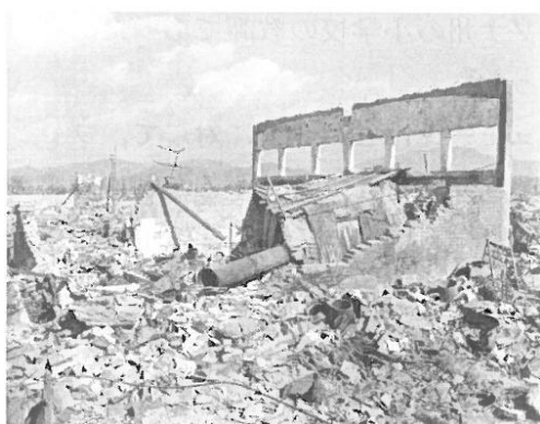
4 Barracks built using a part of collapsed building November 4, 1945 1,320m from hypocenter Sendamachi 1 chome
